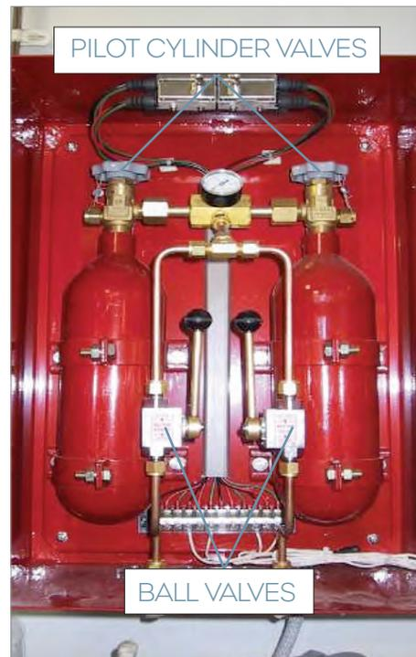
A typical arrangement to control the release of CO<sub>2</sub> into a designated space. In this arrangement, there are only two ball valves. In some systems up to four ball valves may be required.
