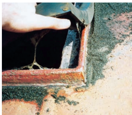
Fig. 26. Example of a temporary rubber attached to the compression bar to compensate for worn seal rubber
