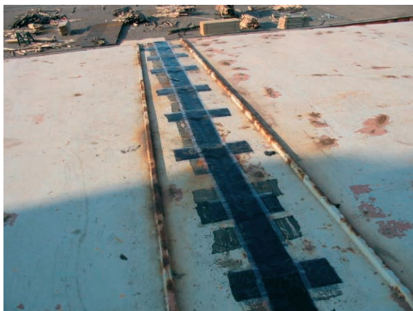
Fig. 35. Example of application of sealing tape to a cross-joint
