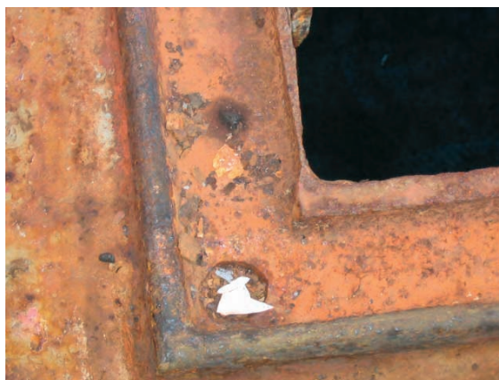
Fig. 23. Blocked drain
