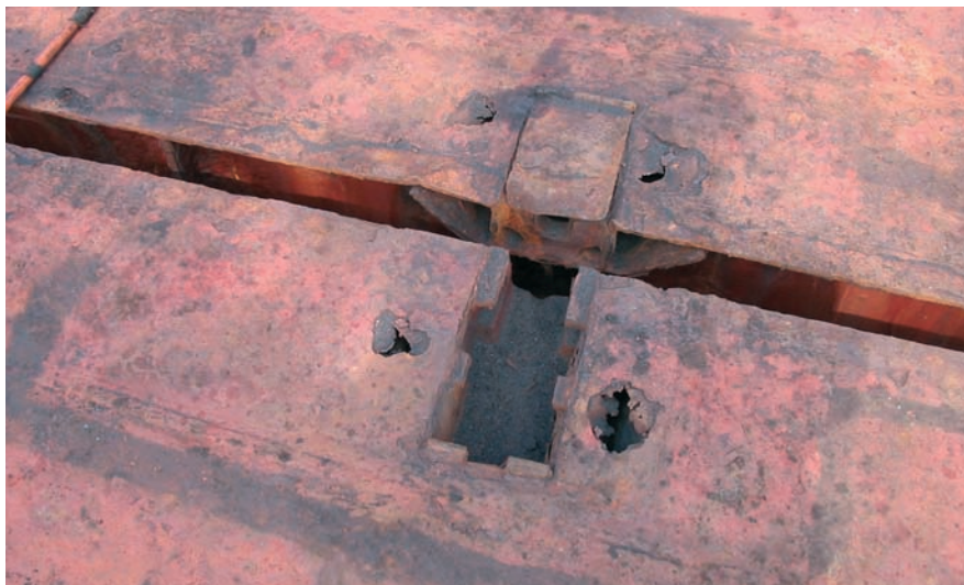
Fig. 30. Localised severe corrosion
