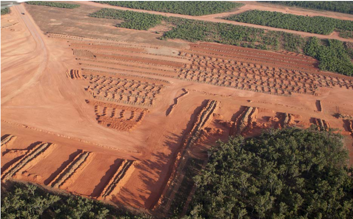
Figure 11 – Australian bauxite mine
