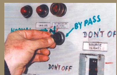
Key operated limit switch
